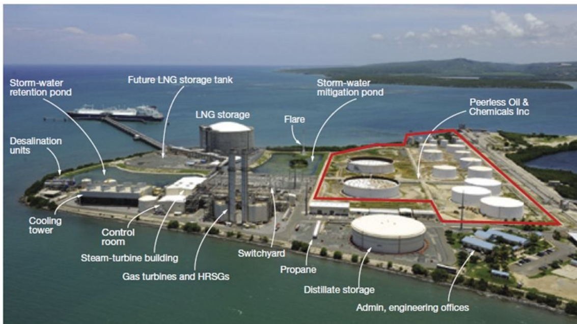
1. EcoElectrica shares a small peninsula with Peerless Oil & Chemicals Inc that juts out into Guayanilla Bay and the Caribbean Sea beyond. Here an LNG tanker discharges its cargo to the 1-million-bbl storage tank via a pipeline mounted on the causeway connecting the plant site to the unloading dock
